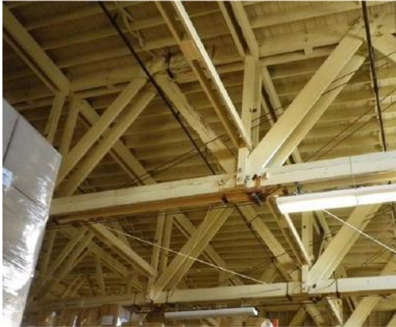
Figure 5: 34m long double-span Warren Truss
