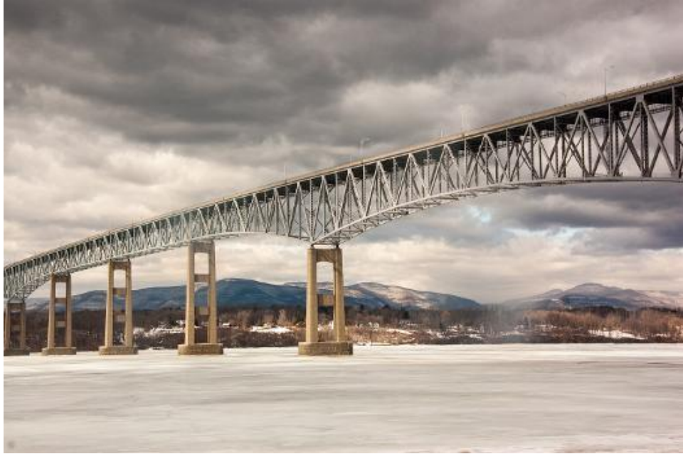
Figure 2-1: Kingston Rhinecliff Bridge
