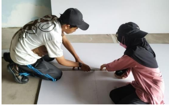
(a) Cutting the gypsum board
