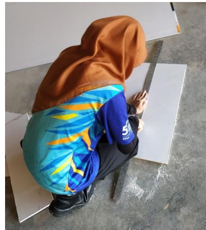
Cutting the board to specified
