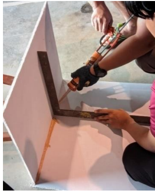
(b) Apply the construction sealant
