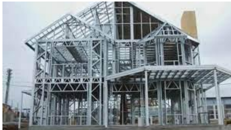
Figure 1.1 Example building made up from the CFS
