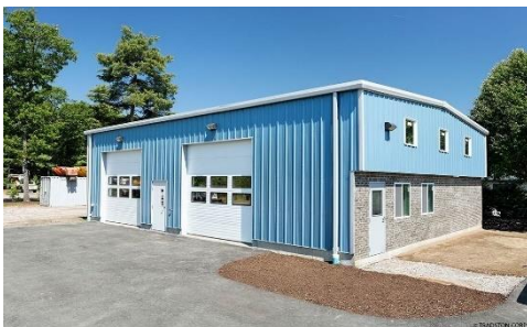
(a) Commercial Building
