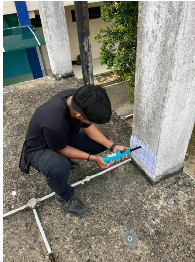
Figure 3.11 Rebound hammer testing (horizontal) on the column
