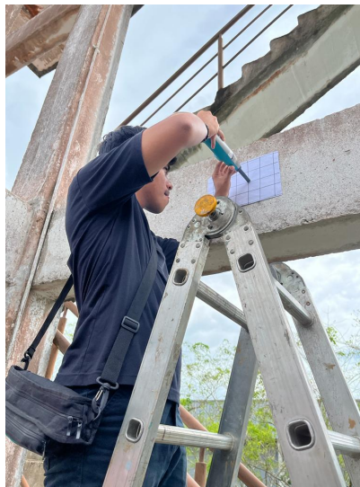
Figure 3.12 Rebound hammer testing (horizontal) on the beam
