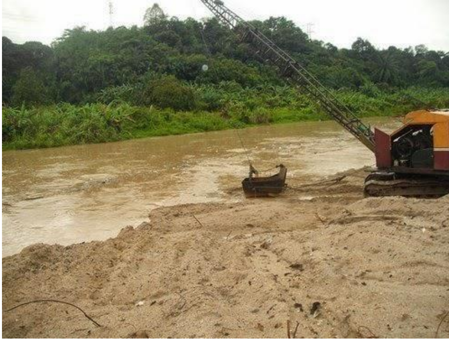
Figure 4.8 : River dredging activities in Sg. Galing, Kuantan
