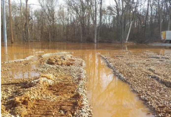
Figure 2.16 : Grading along Maryville Pike in Knoxville pumped sediment into a nearby stream and on to the Tennessee River (Tennessee Lookout,2013)
