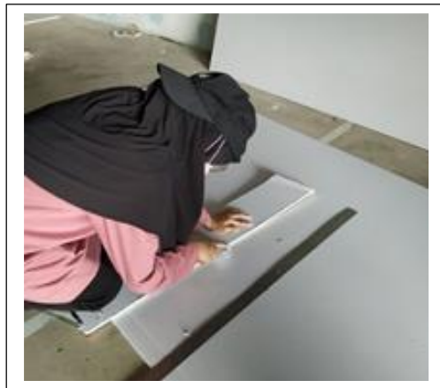
Cut the gypsum board
