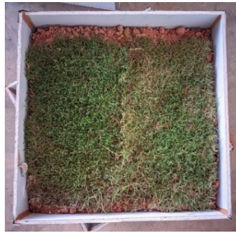
Figure 3.14 Vegetation layer of the green roof (Philippine Grass)
