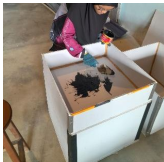
Figure 3.10 Process of applying the bitumen sealant at the bottom of the structure
