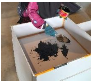
Figure 3.22 Application of bitumen sealant
