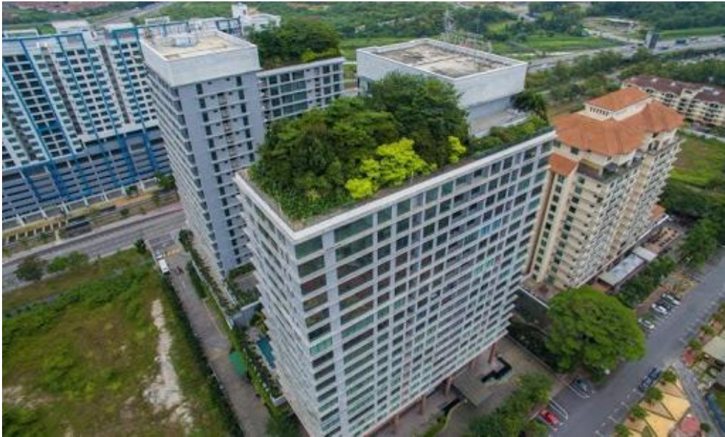
Figure 2.4 Intensive Green Roofs at Acappella Residence, Shah Alam
