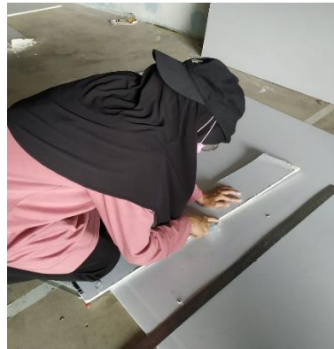
Figure 3.6 Process of cutting gypsum board
