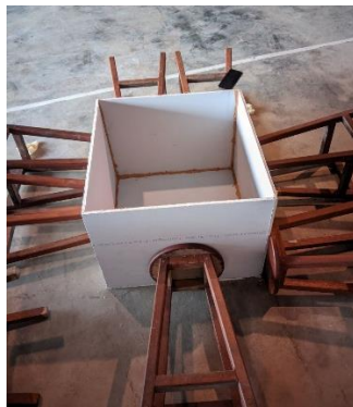
Figure 3.8 Let the construction sealant completely dry
