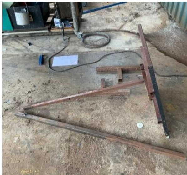
Figure 3.7 Fabrication of Solar Mounting
