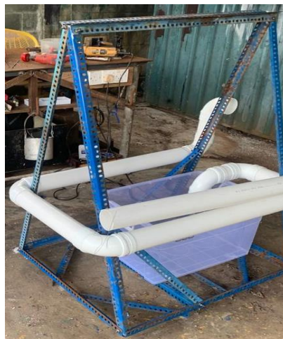
Figure 3.5 Completed Main Structure after fabrication
