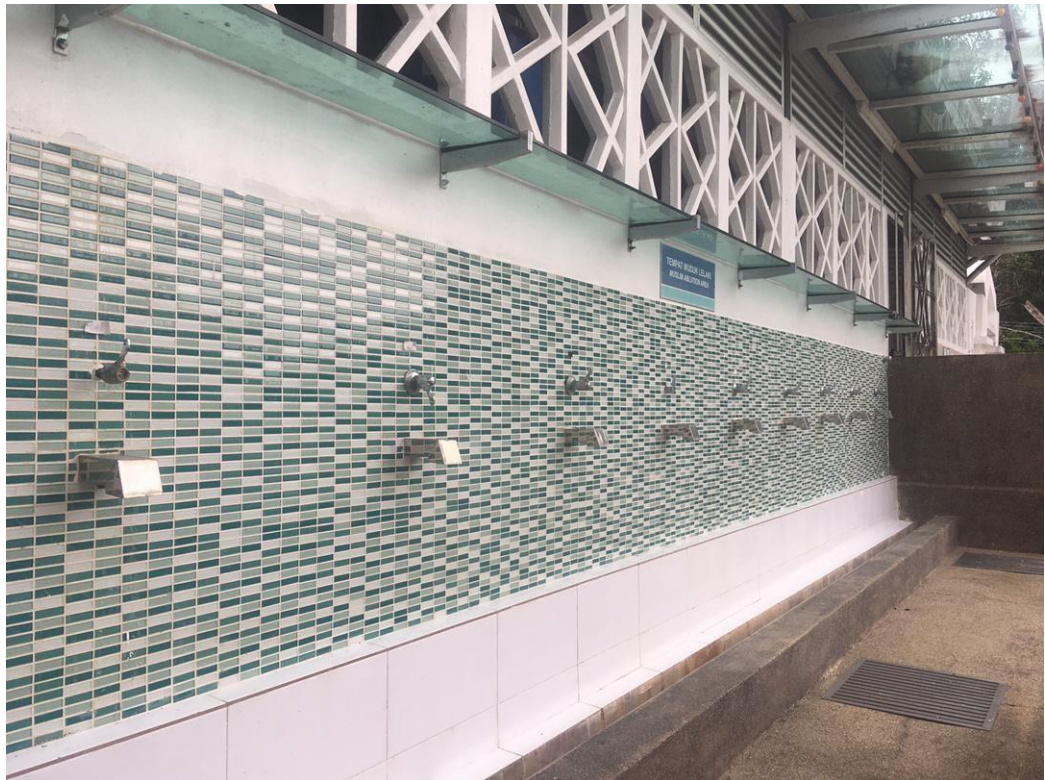
Figure 3.4(b): Outdoor Ablution Area of UMP Gambang Mosque
