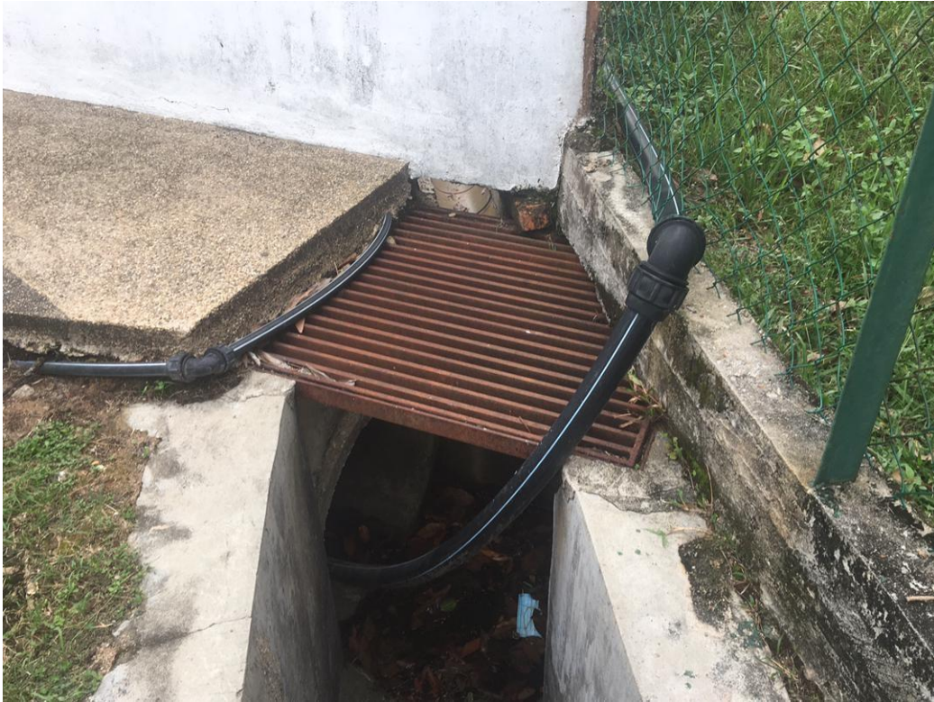
Figure 3.4(c): Discharge Outlet of UMP Gombang Mosque
