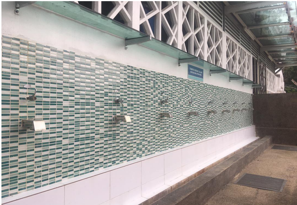
Figure 3.4(b): Outdoor Ablution Area of UMP Gambang Mosque
