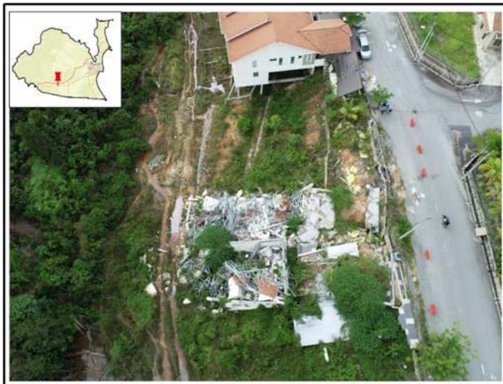
Figure 4: Top view of landslide event at Taman Gambang Damai, Kuantan. This image was captured using drone DJI GL6D10A.
