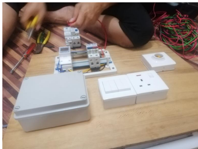
Figure 3.15 Installing main switch, ELCB and MCB
