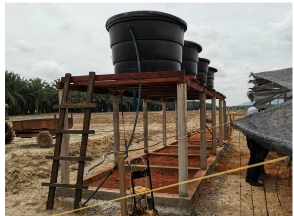
Figure D8 Water Tank in Pre-Nursery
