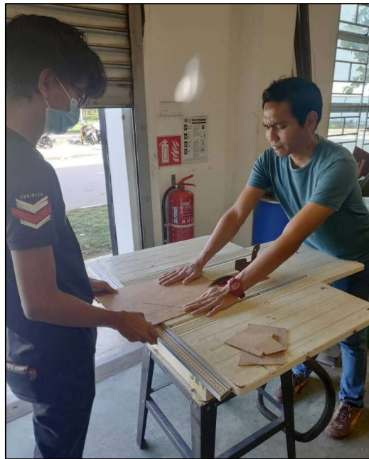
Figure 3.37: Cutting process for front side of boat
