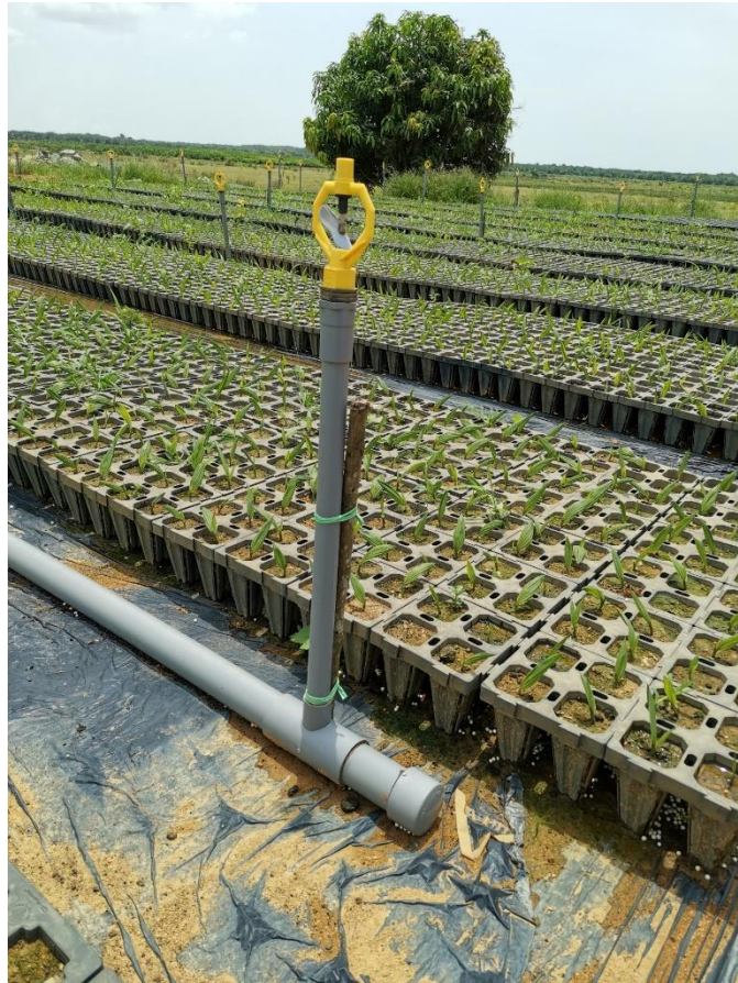
Sprinkler system at pre-nursery
