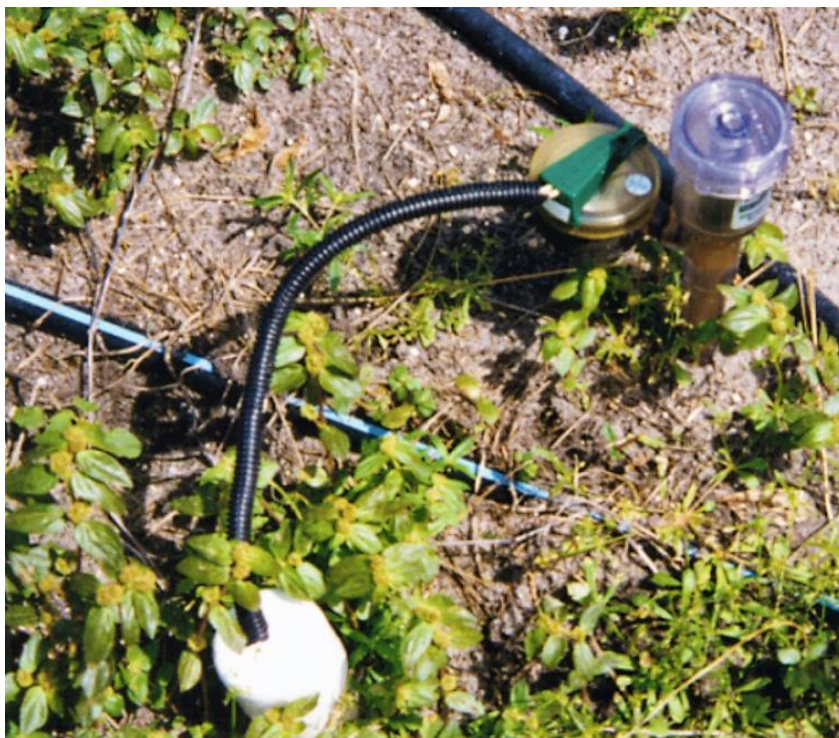
Figure 2.4 A simple version of a closed loop control system is that of an irrigation controller.
