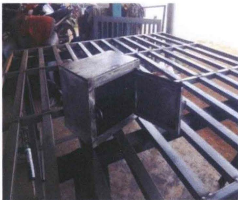
Figure 18 The welding result of Basement of the SSWT
