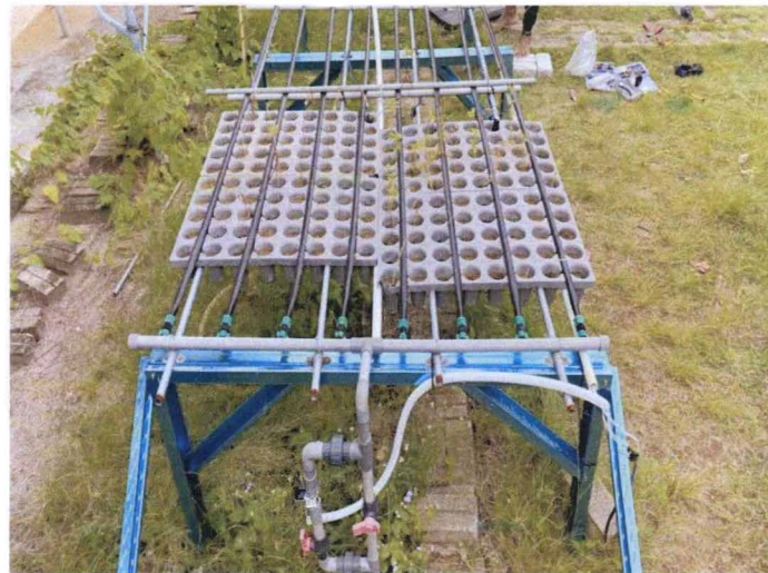
Figure 3.4 Piping System & Valve
