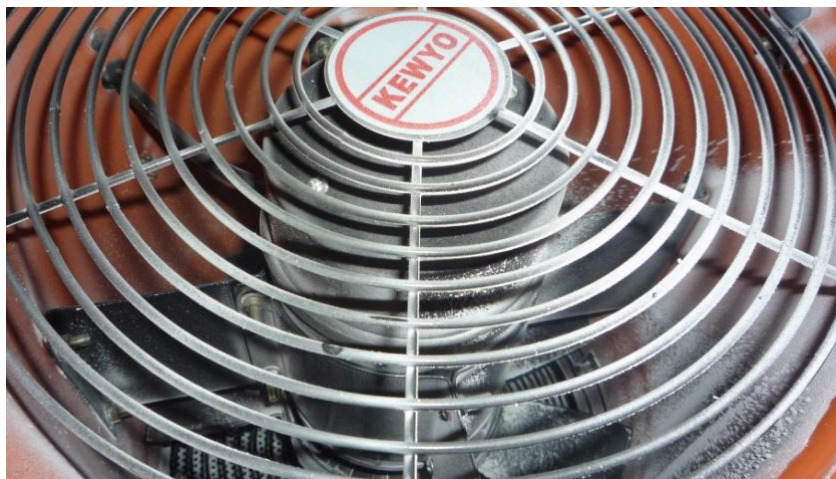
Figure 4.24: ZnO stuck at the exhaust fan
