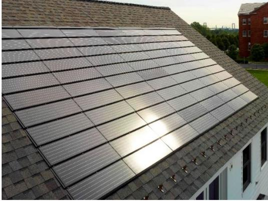
Figure 2.2 Building integrated photovoltaics (BIPV)
