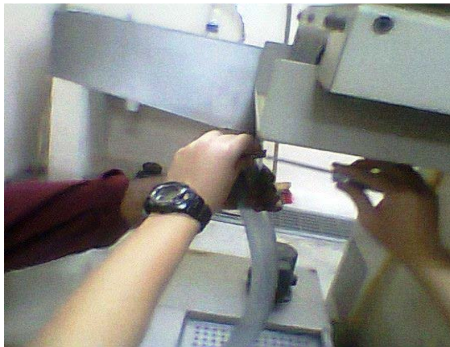
Figure 3.10: Nanocoolant pipe fixing
