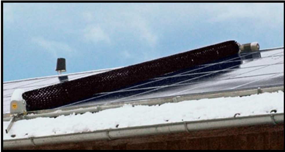
Figure 2.7: PV panel with automatic cleaning system
