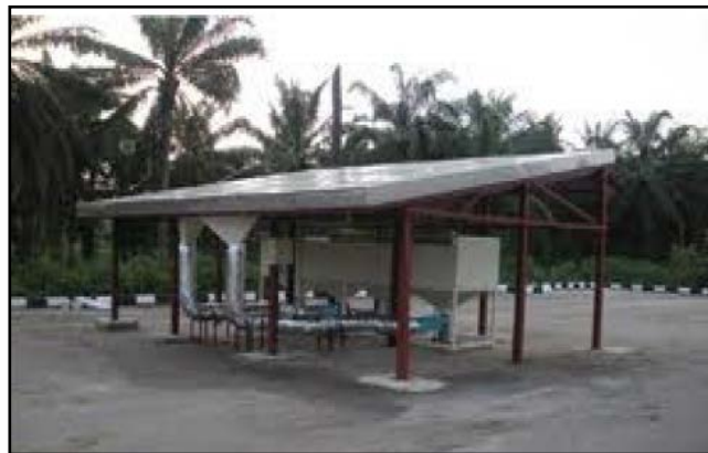
Figure 2.10: Photograph of solar drying system
