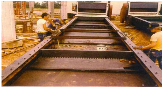
Figure 2.15: Screening process unit
