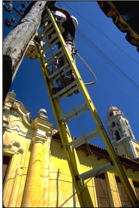
Figure 2.6: Work using the ladder ( http://en.wikipedia.org/wiki/Ladder )
