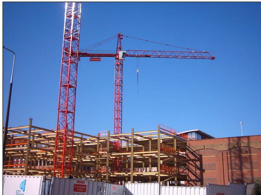
Figure 2.8: Crane operation in the construction site ( http://thecrane.com.my/ )
