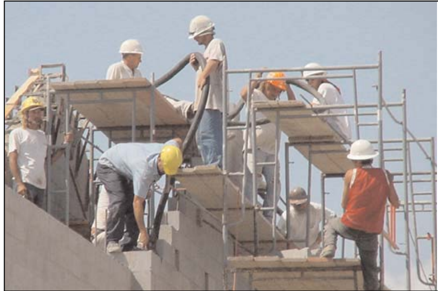
Figure 2.4: Work using Scaffolding ( http://en.wikipedia.org/wiki/Scaffolding )
