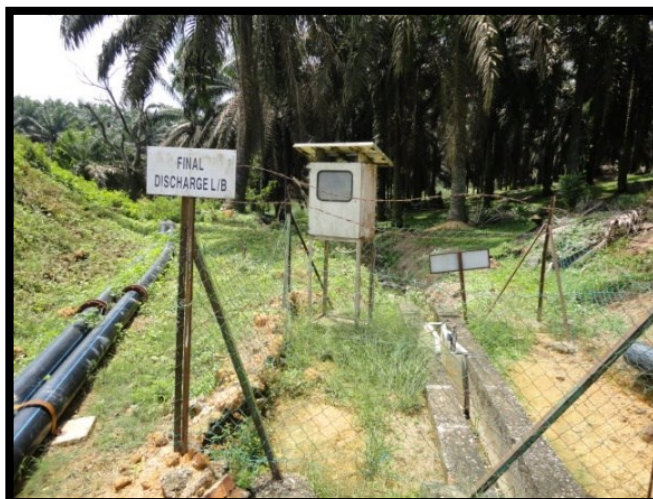
Figure 3.2: final effluent discharge by watercourse
