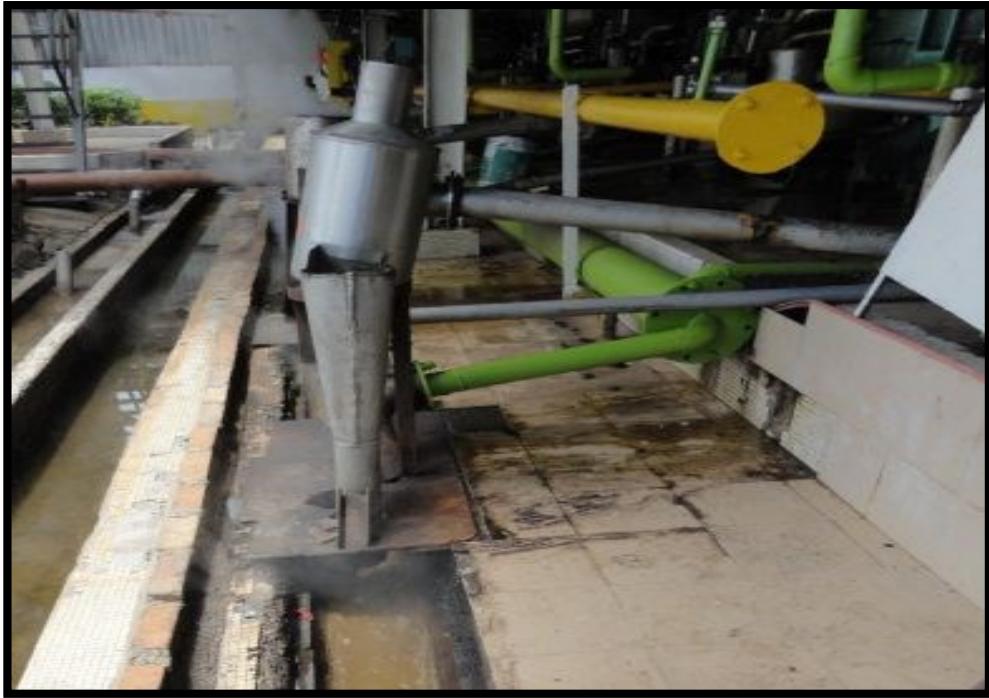
Figure 2.1: Fresh POME discharge from plant.
