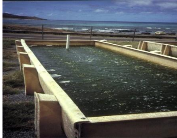
A. Deep Aerated Tank
