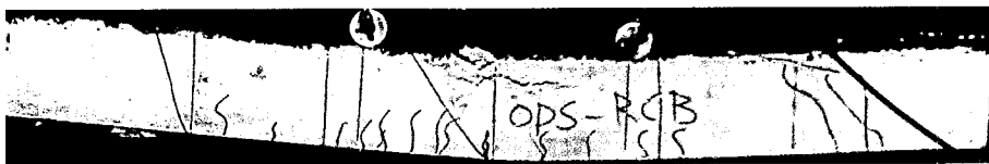
Figure 1 OPS reinforced concrete beam without fibres (Control beam)
