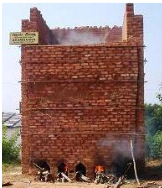
Figure C: Brick and concrete kiln
