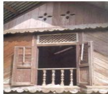
Figure 2.4: Designed to suit the local climatic requirements using various ventilation and solar control devices, and low thermal capacity building materials
