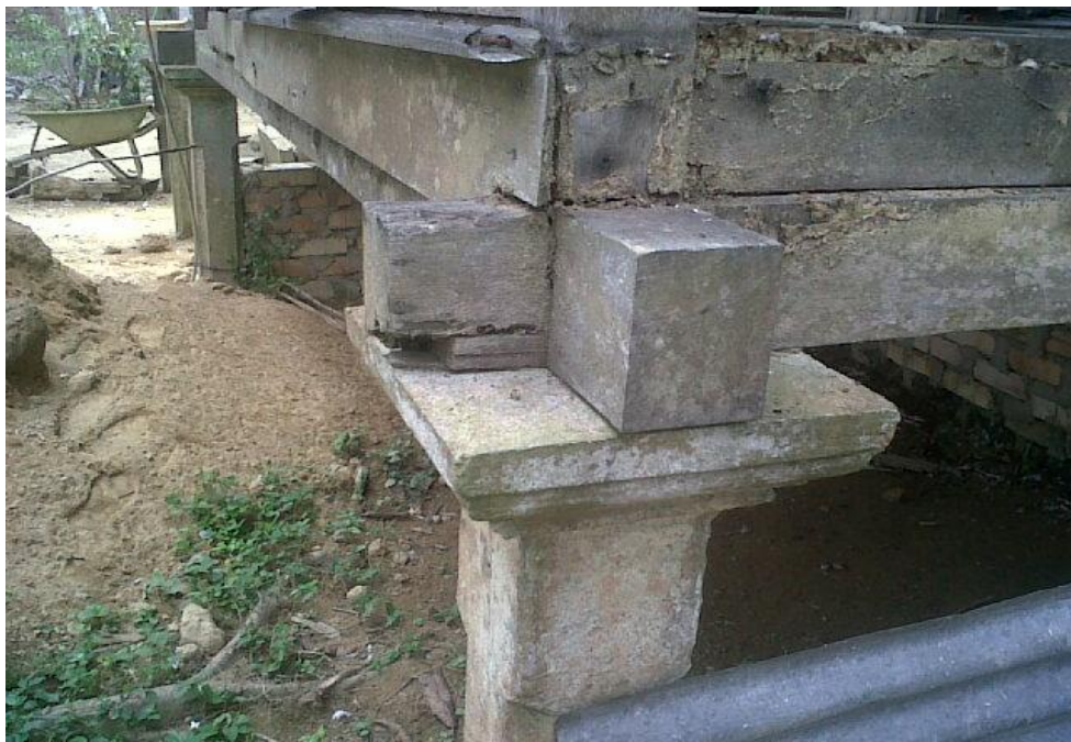
Figure 3.3a: The column the front of the house
