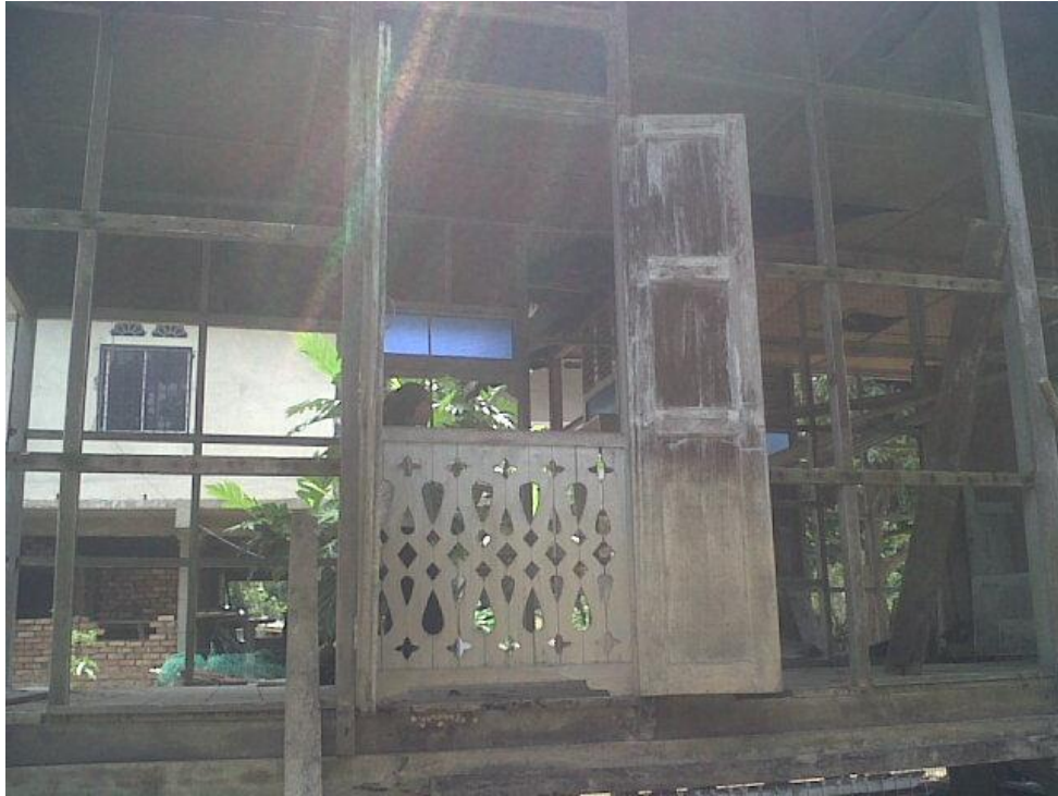
Figure 3.2b: The window (window panel opened)
