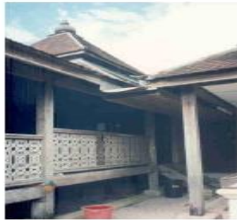
Figure 2.4: Designed to suit the local climatic requirements using various ventilation and solar control devices, and low thermal capacity building materials
