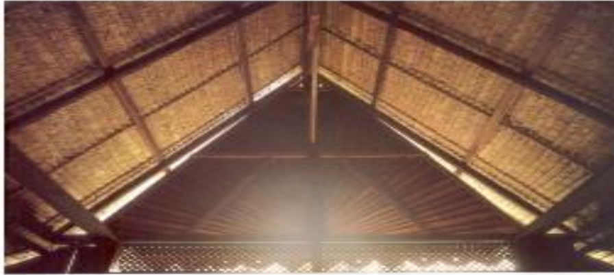
Figure 2.3: Steep roof and openings allows for fast water runoffs and facilitates circulation of hot air out of the house to increase natural ventilation.
