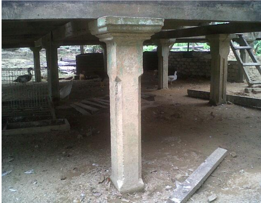
Figure 3.3b: The column at the back of the house
