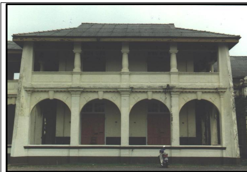
Figure 3.2: High School Muar building
