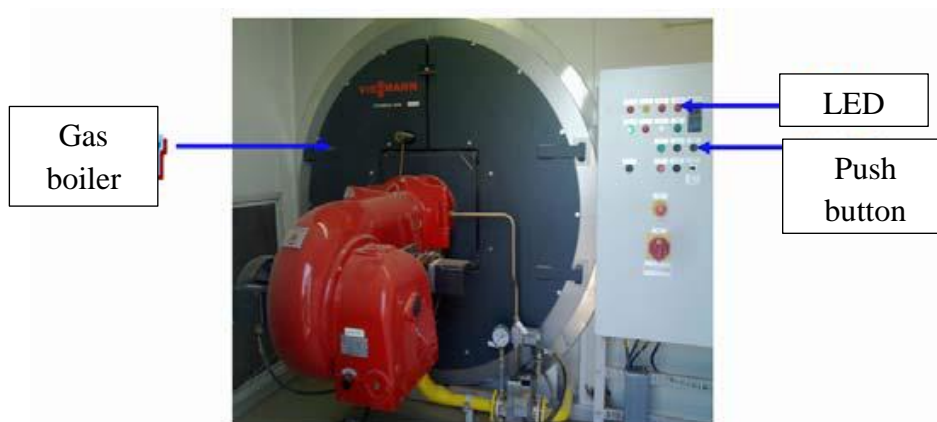
Figure 2.10: Local control panel of GRS
