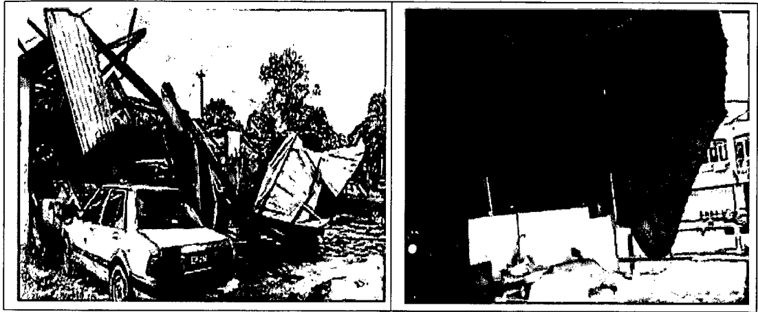
Figure 1.2 Damage Roof (Berita Harian, 2011)
