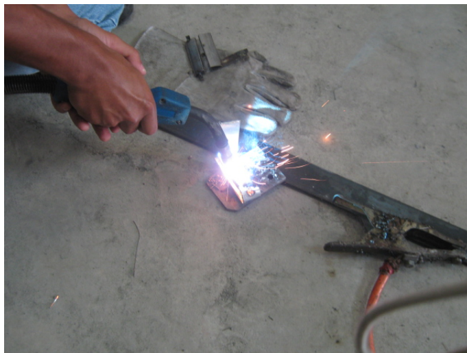
Figure 4.10: Welding Process by using MIG weld type
