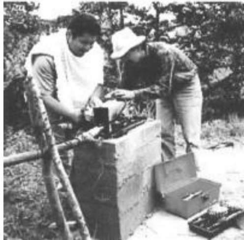
Figure 2.9: A Colombian manufacturer installing a DC Pico-Hydro Generation system (Source: Lahimer, 2011)
