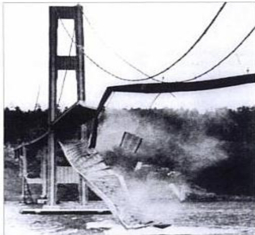
Figure 1.1: Tacoma bridge failure
