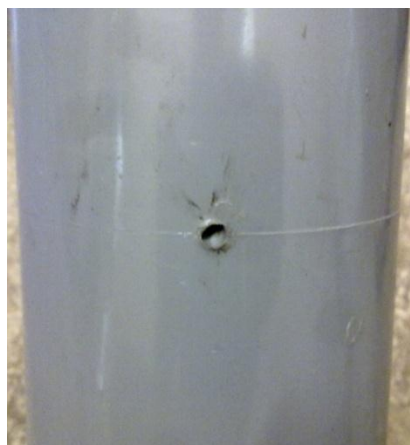
Figure 3.13 (2 mm) defect introduced on tee
