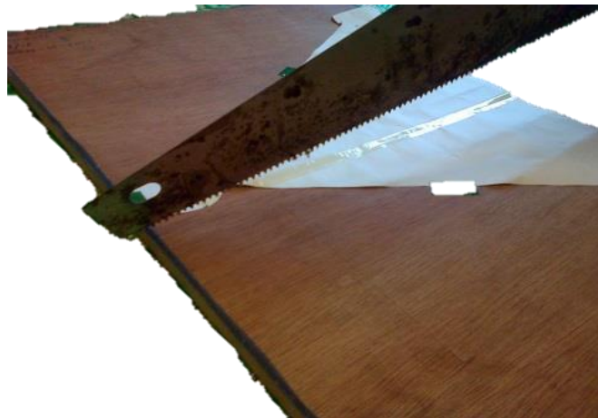
Figure 3.14: Cutting the softboard with Jig-saw
