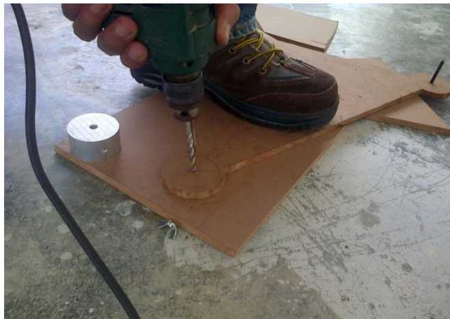
Figure 3.15: Drill the holes with hand drill
