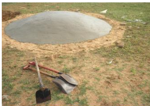
Figure 3.21: Roof Mould
