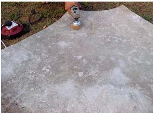
Figure 3.22: Roof after Cutting Process
