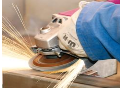
Figure 3.14: Clean roughness surface area by using Grinding Machine.
