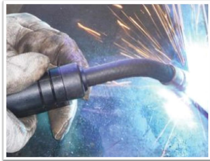
Figure 3.11: Welding Process Using MIG Welding
