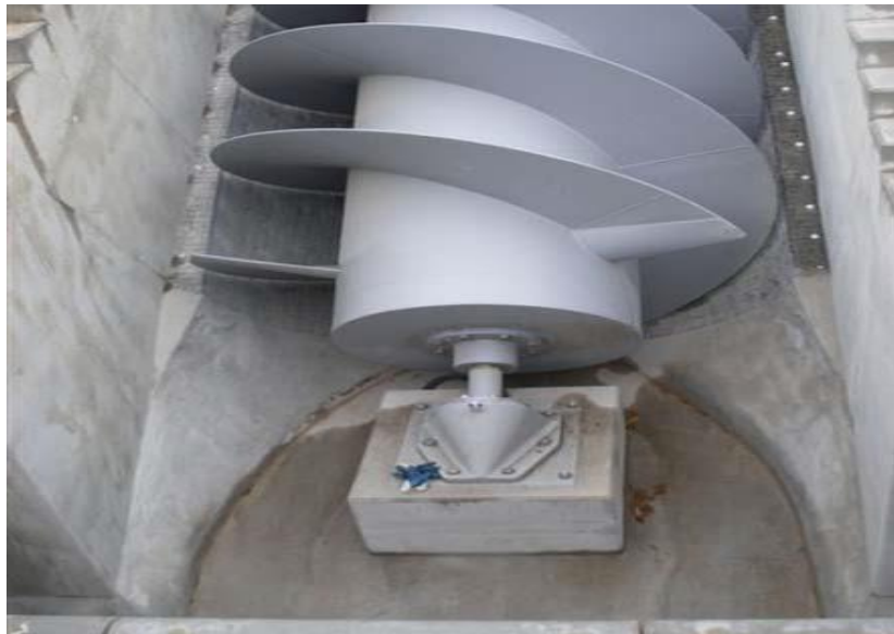
Figure 2.3 : Concrete Trough
