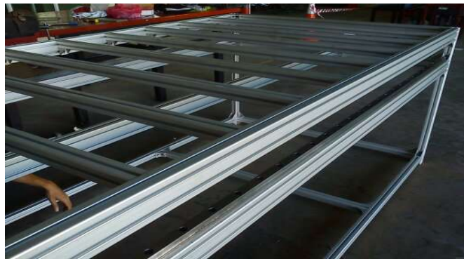
Figure 17: Addition part of the structure.
