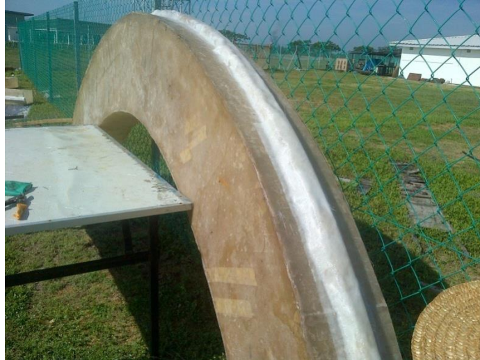
Figure 4.7(c): The reinforcement is assembled together the curve tank.
