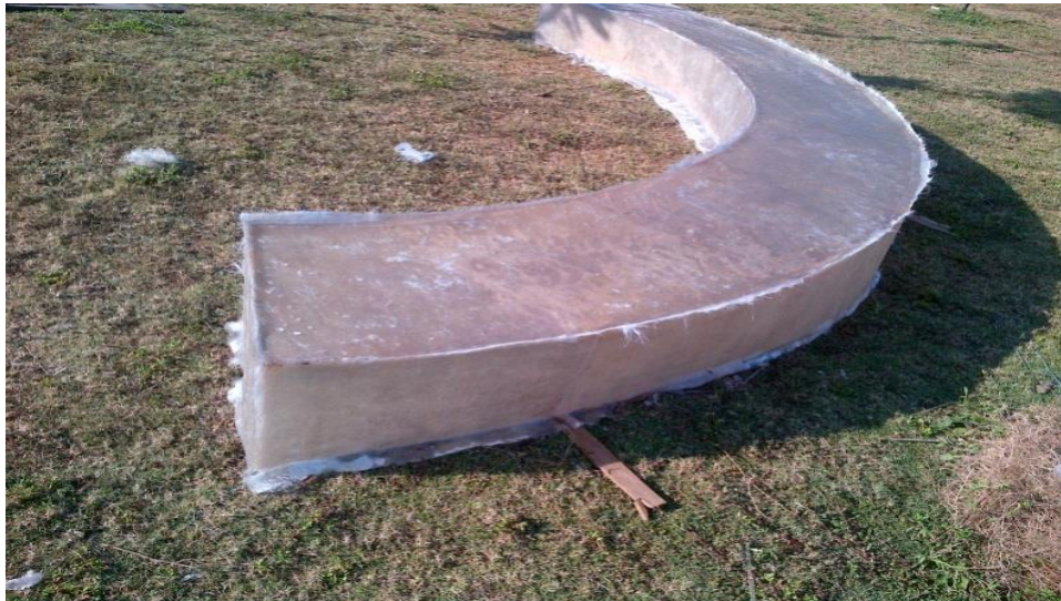
Figure 4.4: The fabrication of curved tank
