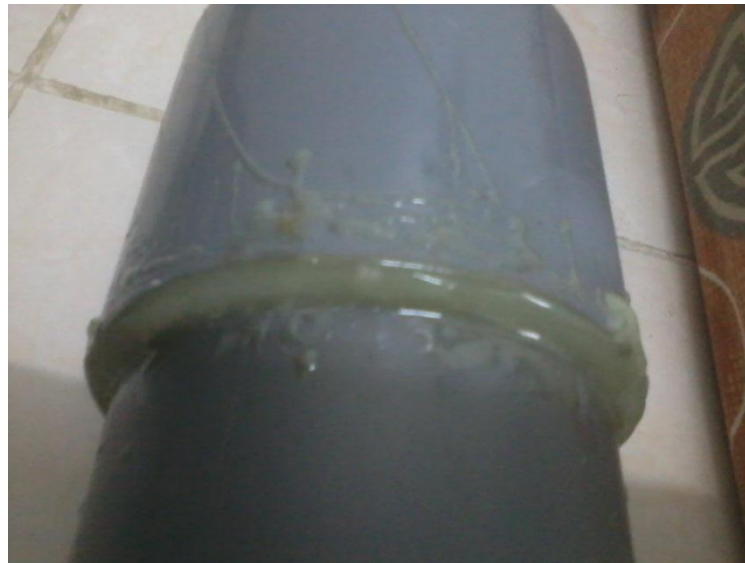
Figure 4.6: Application of Araldite Epoxy at the joint
