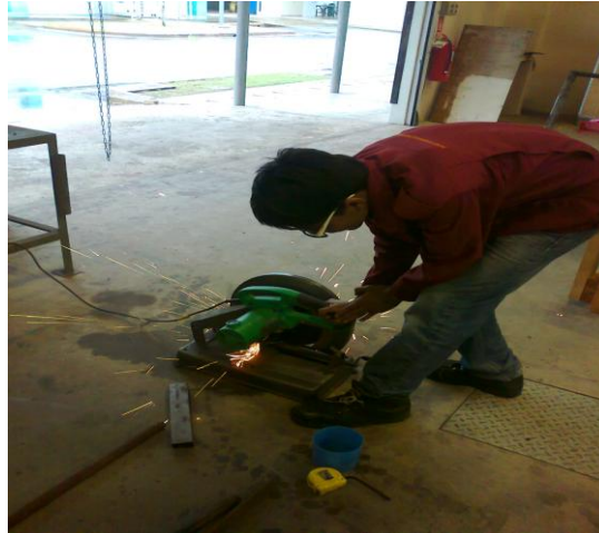
Figure 4.2: Cuts Materials using Floor Cutting Disc Machine
