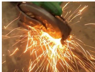
Figure 4.4 : Cutting Process started
