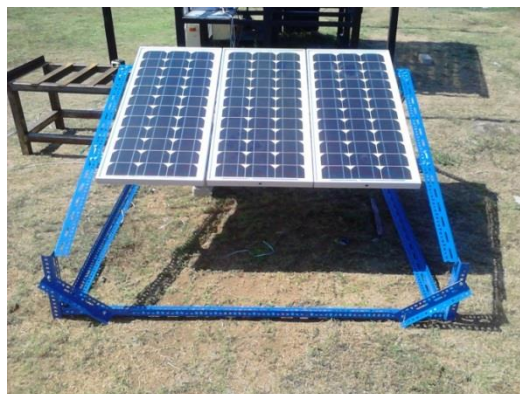
Figure 4.8: Test Rig of Solar Panel Used
