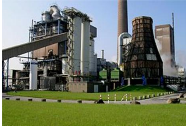
Figure 1.1: Oldest power station utilizing circular fluidized bed technology, in Lünen, Germany country.
