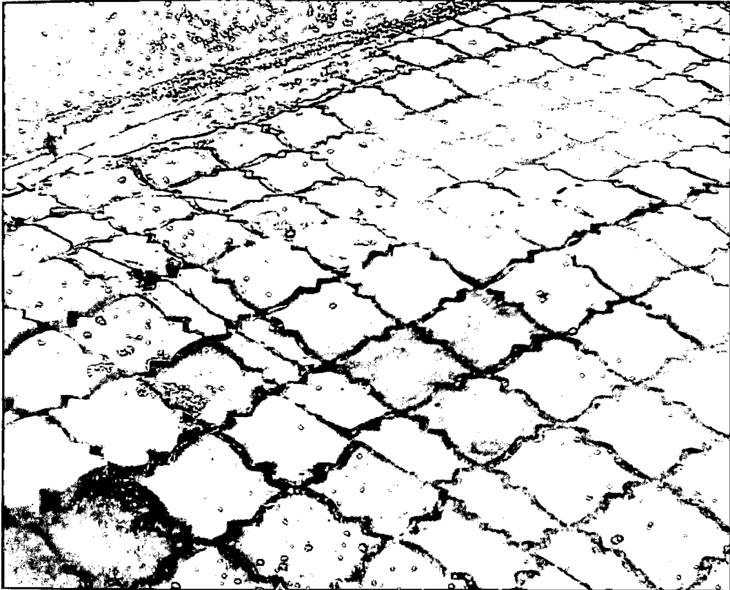
Figure 1.1: Defect on walkway
