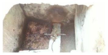
Fig. 3. Flowmeter sensor fixed to bottom of sewer pipe
